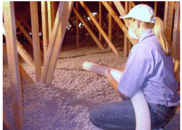
Installing loose-fill cellulose in an attic.
