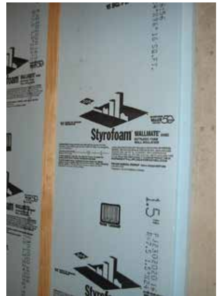
Rigid foam against a foundation.
